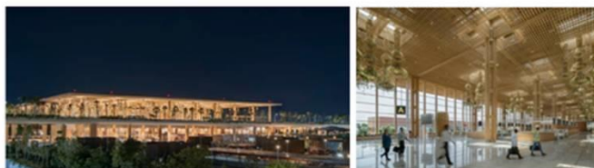
Figure 6: Terminal 2 Kempegowda International Airport, Bengaluru, India
