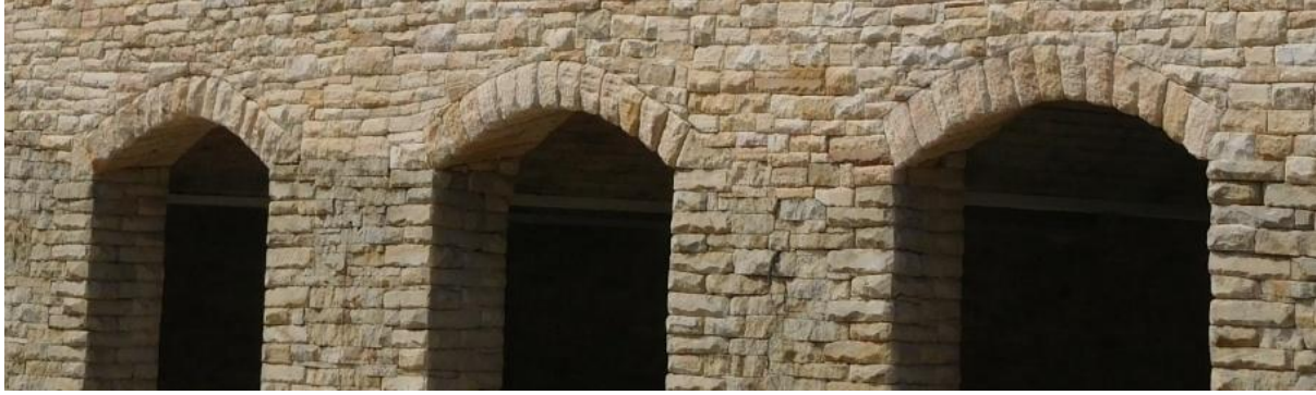
Arches are curved vertical cladding, spanning an open space beneath. It supports the stones above. Ray house, Alibag
