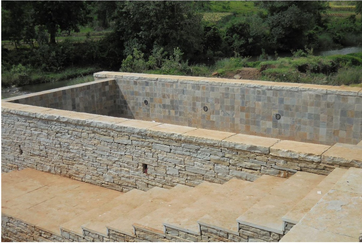
Wall caps, use self-weight to lock the wall stones beneath – making them self-sustainable.
