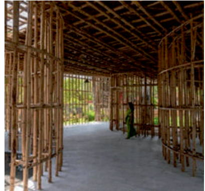
FIG.3 North-East Pavilion, Surajkund Lake, Faridabad by AT Architecture, Mumbai (Dezeen, n.d.)
