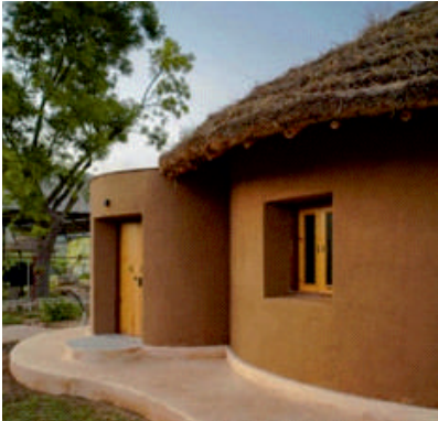
India. FIG.2 Gol Ghar, Rajasthan by Sketch Design Studio (Sketch Design Studio, 2014)
